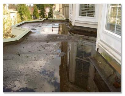
There is evidence of a lot of moisture at the soffit panels, below some of the first floor portico roofs. Most likely this is coming from water entering via a failed roof membrane above.
