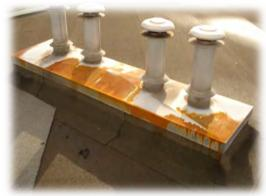
There are clear signs of wear to the overall area of the roof including: little or no cover-gravel remaining, top layer of the membrane cracking, seams gapping, membrane lifting and ridging and membrane soft-spots.
