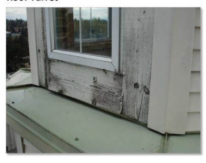
The roof has a decorative turret made up of windows, window trim and siding, with typical flashings and weather trim. The turret did not have the benefit of the window remediation conducted on the rest of the building a decade earlier. This enables us to see the effects of the weathering that the earlier remediation efforts prevented. It should be noted, this was constructed under building practices typical of the 1995 condo building era.
