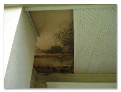
One of the most troubling findings was heavy mold and mildew growth due to excessive moisture in some of the deck soffits.
