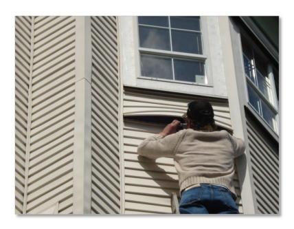
For the most part the siding was performing as expected. There are a few locations where the siding has come unattached, is slipping and needs to be re-attached. Considerable care should be taken to ensure the same pieces of siding can be re-installed. If the old siding needs to be replaced, a close match may be difficult to acquire.
