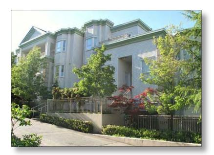
The Condominium consists of three buildings, the larger condominium building at [ ] Ave., consists of 108-unit condominium building contained within a four story wood framed structure built on a concrete parking garage. The building is generally rectangular in shape with two courtyards on the north side of the building. There are two townhouse buildings the first at [ ] Ave consisting of 14-
