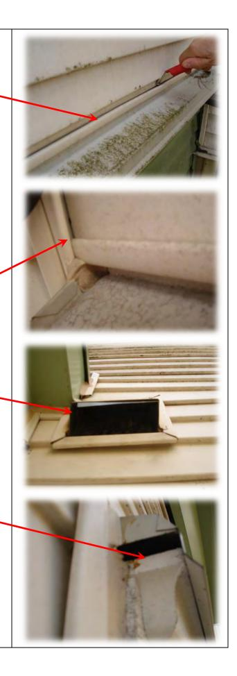
SW Side: Siding and trim details at junction points were inadequate in numerous locations. In a number of locations on all buildings there are gaps where water can gain access behind the siding leaving only the building paper as the defense against water.
