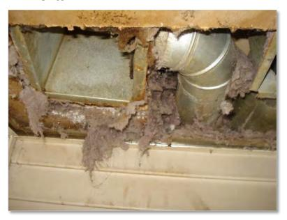
Some of the venting systems that exhaust moist air from inside the living spaces are a concern. Lint accumulation and moisture retention were noted in more than one location and in some, the lint buildup is so severe, we question whether there is any lint filtration for the clothes dryer at all. And, to exacerbate the problem, many of those air vents are channeled to exit through the patio deck ceilings, which, as mentioned earlier, are poorly ventilated,
