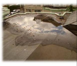
Seams between the bitumen rolls are dried out and many are brittle enough to begin breaking off making the seams vulnerable to water ingress beneath the membrane.
