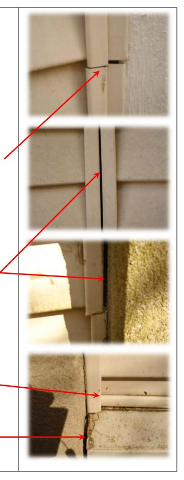
SW Side: In a number of locations on all buildings, shrinkage of the building has caused the Hurricane ties, which are attached under the siding, to bow putting outward pressure on the siding and pushing it out. This creates "bumps" in the siding and in some cases has caused the siding to detach. Our recommendation is to send a work team around the building(s) to repair hurricane strap deficiencies using best-practice siding installation techniques
