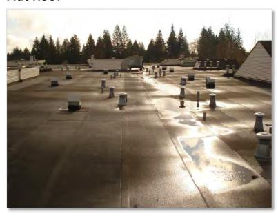
The roof appears to be well maintained. One of the first impressions is how clean and clear of debris the roof is. But, the roof is aging and close to end of life. We estimate 15% of the flat-roof has been patched to date, not unexpected on a roof now 17-18 years old.
