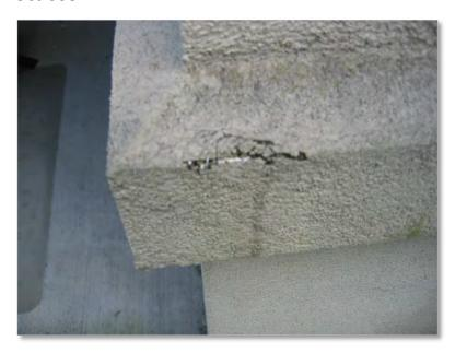
In a number of locations the protective stucco membrane has been broken allowing water to access the internal structural components.
