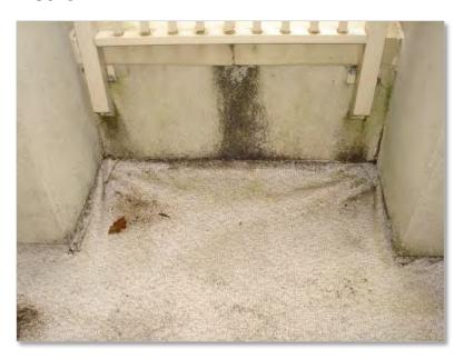
Some decks were quite dirty with mold accumulating and jeopardizing the health of the deck floor membrane.
